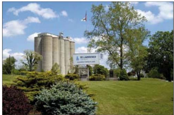
Figure 1 St Lawrence Cement's Hagerstown plant.
