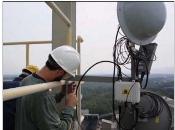
Figure 2 Installation of sector antennas and wireless router.
