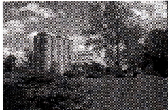
Figure 1 St Lawrence Cement's Hagerstown plant.
